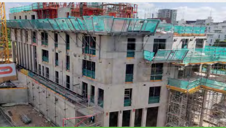
Residential Development Project at Pontoon Dock London, UK (Quelle: Jody Parker, Director at Parker Bromley)
